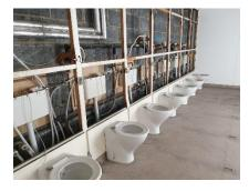
All domestic systems were stripped back to the main incoming pipework to the spaces, and new pipework was installed. DL M&E Building Services also carried out the installation of new sanitaryware consisting of WC pans, WC cisterns, urinals, urinal cisterns, wash basin taps and a stainless-steel sink top.
